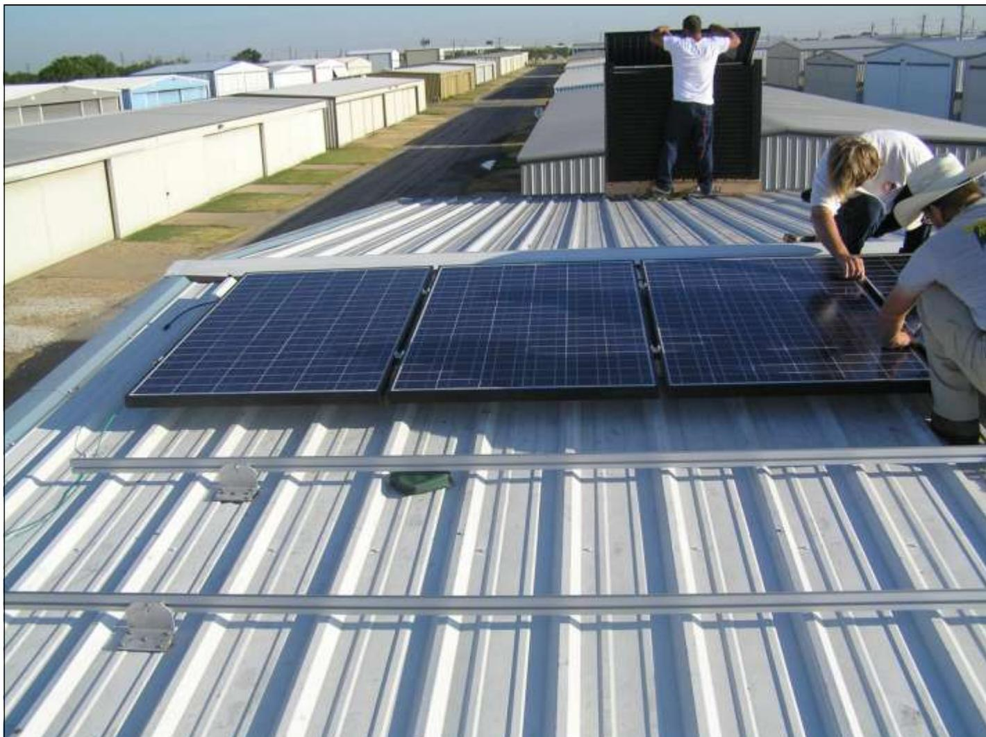
*Workmen spent 3 days installing and wiring the three sets of 18 modules in series.*
