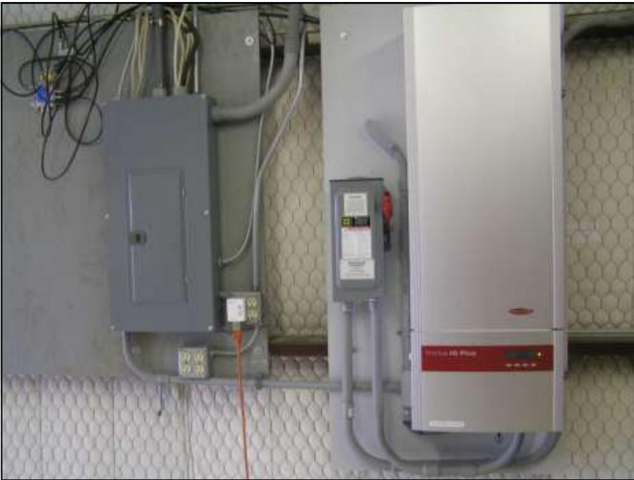
The inverter which converts incoming DC to AC with output reading.
